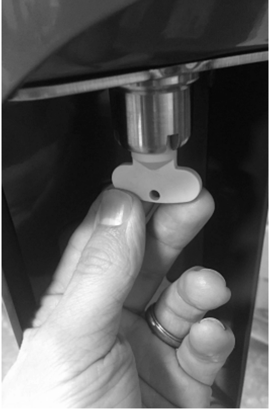
Figure 14: Bottle fill outlet aerator being replaced with aerator key.
