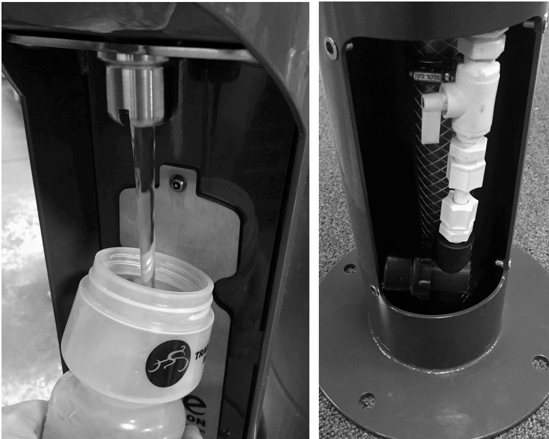
Figure 12: Bottle Fill Station flow adjustment by using the adjustment ball valve.
