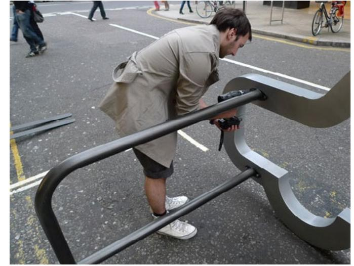
**Step 3:** Take a side rack and place it, lining up the drilled holes. Place 4 x M8 Torx bolt into holes and screw into place using electric drill on low speed. Repeat on the other side.
