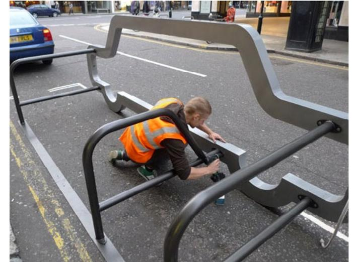
**Step 4:** Take the steel floor plate and place it under the metal rack, lining up the drilled holes. Screw the short M8 Torx bolts into plate. If the holes do not line up, loosen the Torx bolts in the car frame until the holes line up before retightening.
